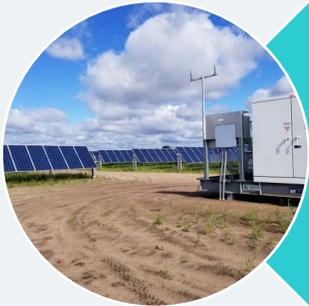
**Invertors:** Central in a solar energy system. It's a device that converts direct current (DC) electricity, which is what a solar panel generates, to alternating current (AC) electricity, which the electrical grid uses.
