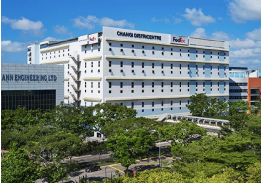
Industrial/Logistics (Warehouse, Factories)
